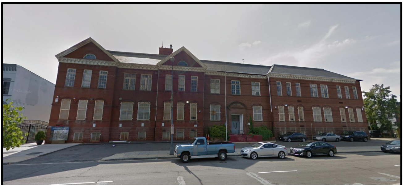
Front façade of the Grimke School
